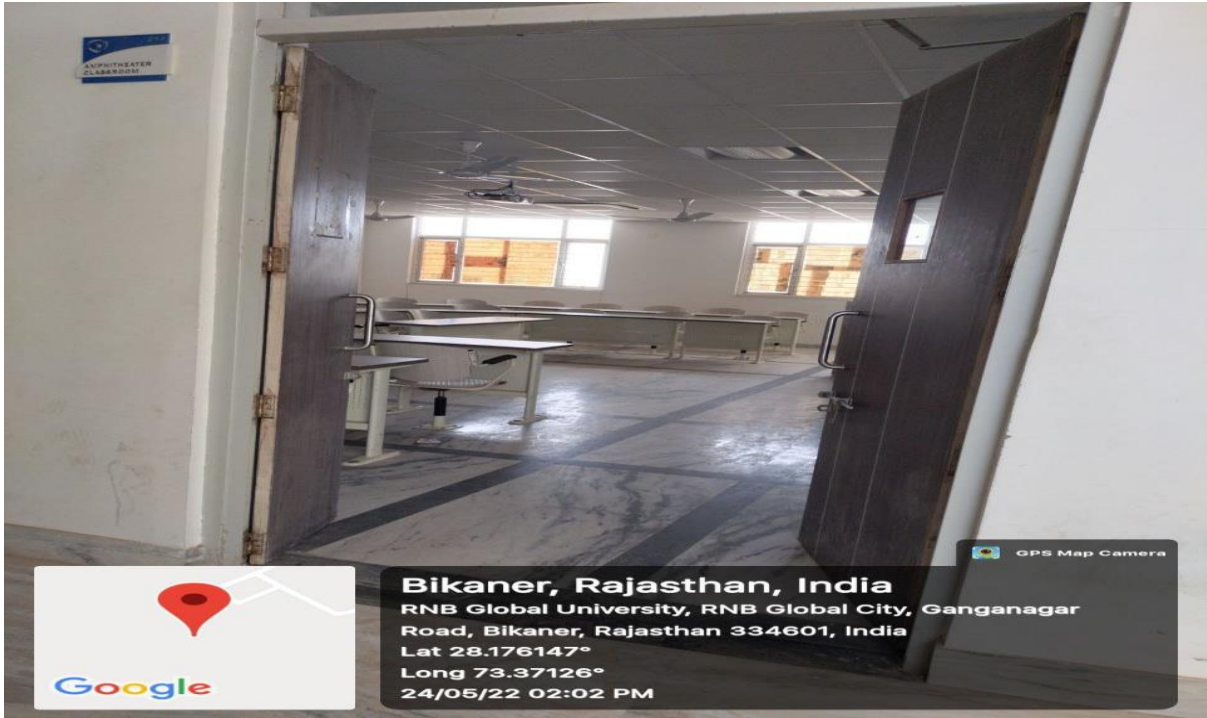
Second Floor Room No. – 213 Classroom front
