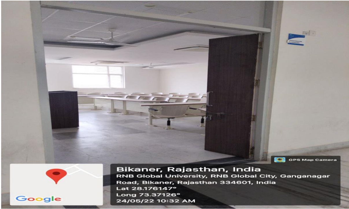
First Floor Room No. 102 Classroom front
